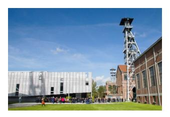
The architects of "Bâtiments de France" demanded that all the facilities to be "reversible", so they can be removed without leaving any traces. The idea consisted in creating "a box in the box" in order to respect the identity of the places.
